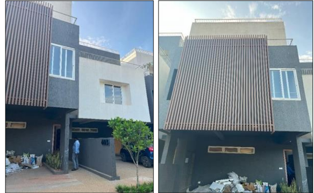
Fig 1 & 2: Exterior view of row house unit 603
